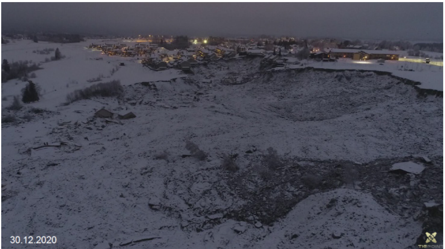
Gjerdrum Quick Clay Landslide, December 2020. Source: Tiepoint AS (Nicholas Newhouse)
